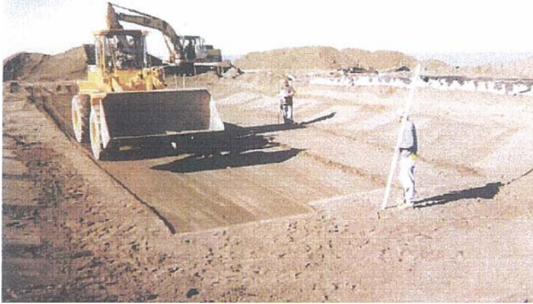
This photo shows the final preparations before liner installation.
